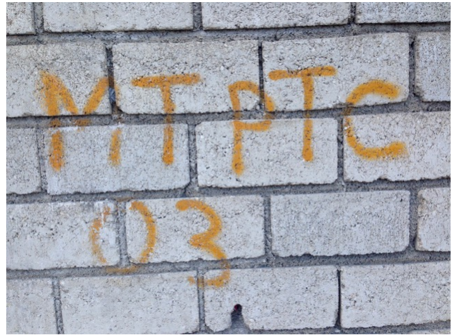
Figure 1: MTPTC paint outside of a Haitian building. The paint color indicates the assessment of the building's structural stability.
